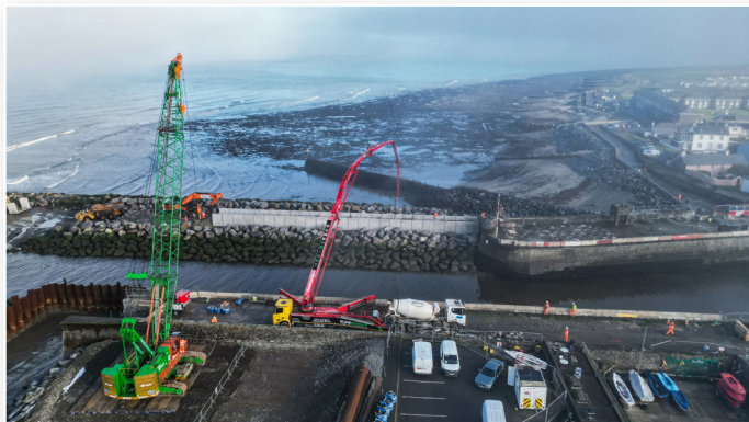
Construction of the North Breakwater concrete walkway
