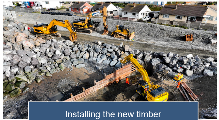
* River Aeron - cladding new reinforced wall with stone
