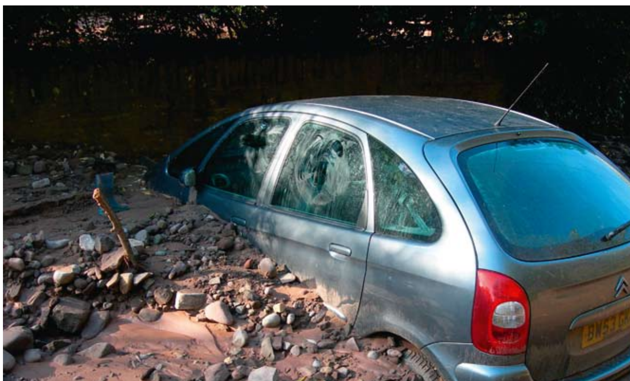
Monmouth and Brecon Canal breach
