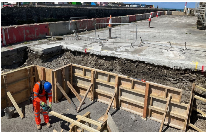
Quay Parade - Formation footing for the replacement wall
