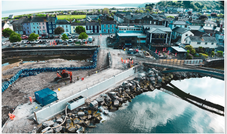
Construction of Pwll Cam terrace wall, ready for masonry cladding and glass panels
