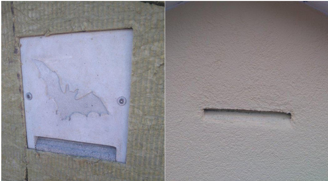
Figure C2- 1: Bat box mitigation/enhancement example
