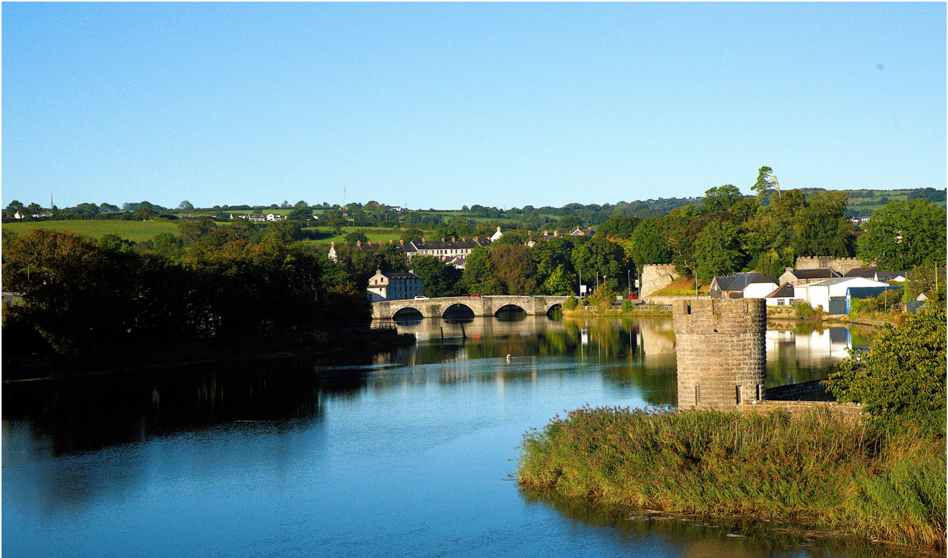
View of the Castle Bridge, image supplied by the Town Council
