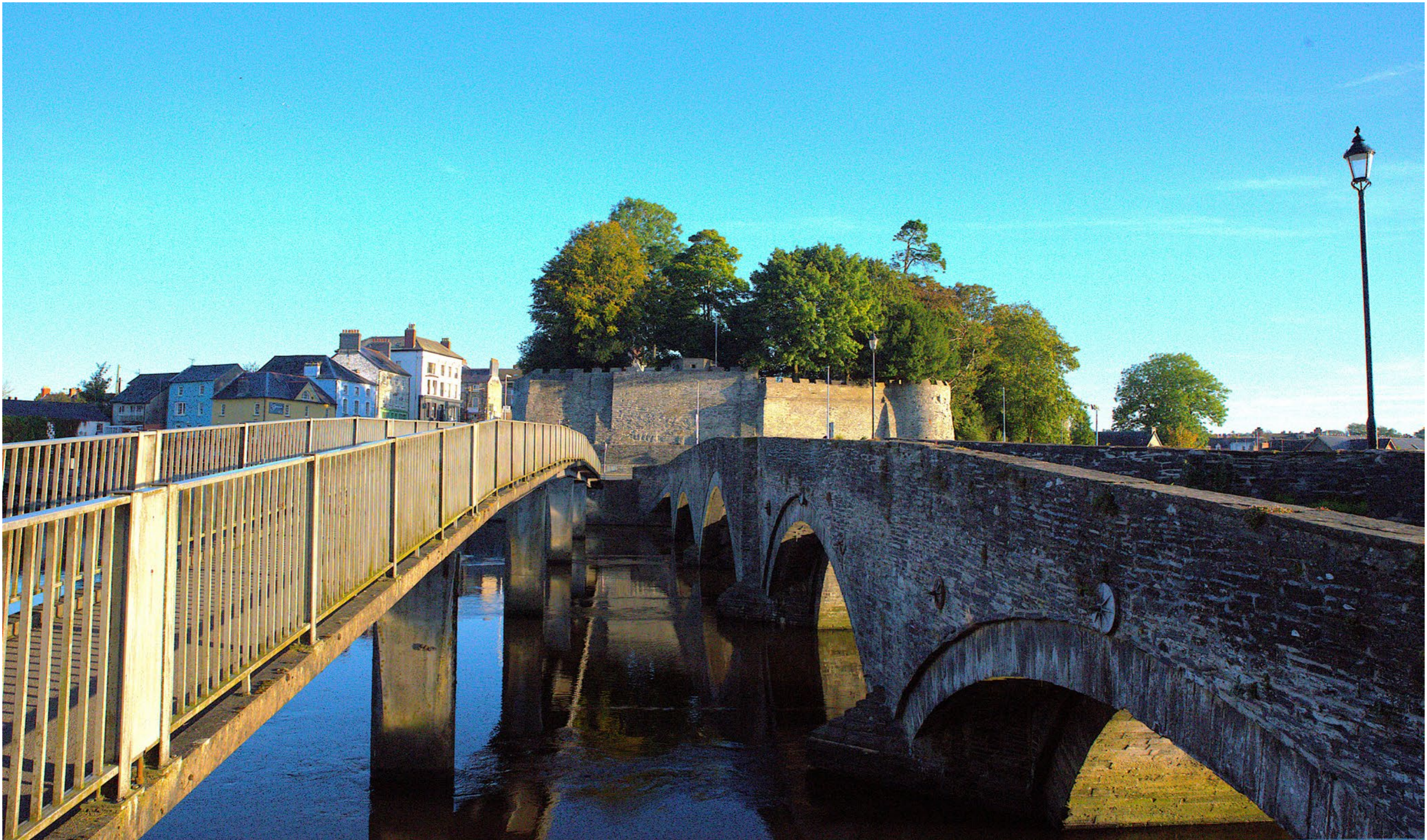
Footbridge and Cardigan Bridge across Afon Teifi, image supplied by the Town Council
