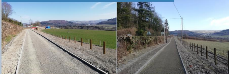
Construction of the new path adjacent to the TRA487
