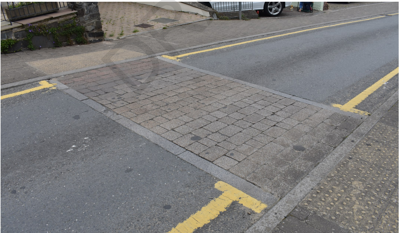
Fig. 10 Careful choice of suitable modern materials and sensitive design, can achieve traffic calming and pedestrian way marking without detracting from the historic character of a place.
