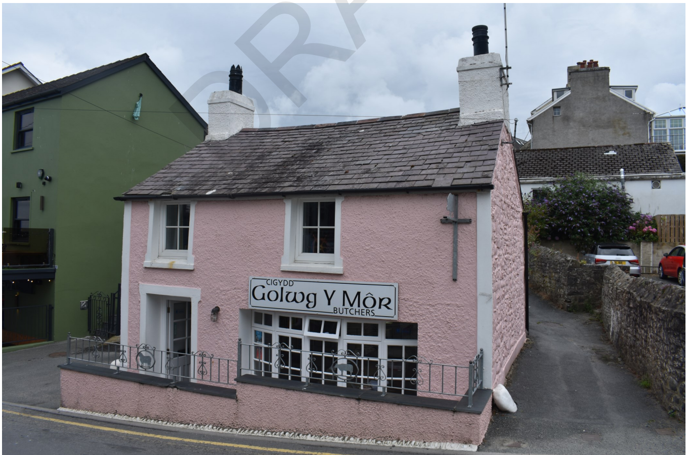
Fig. 6 Warehouses and small stone cottages are remnants of earlier development at New Quay
