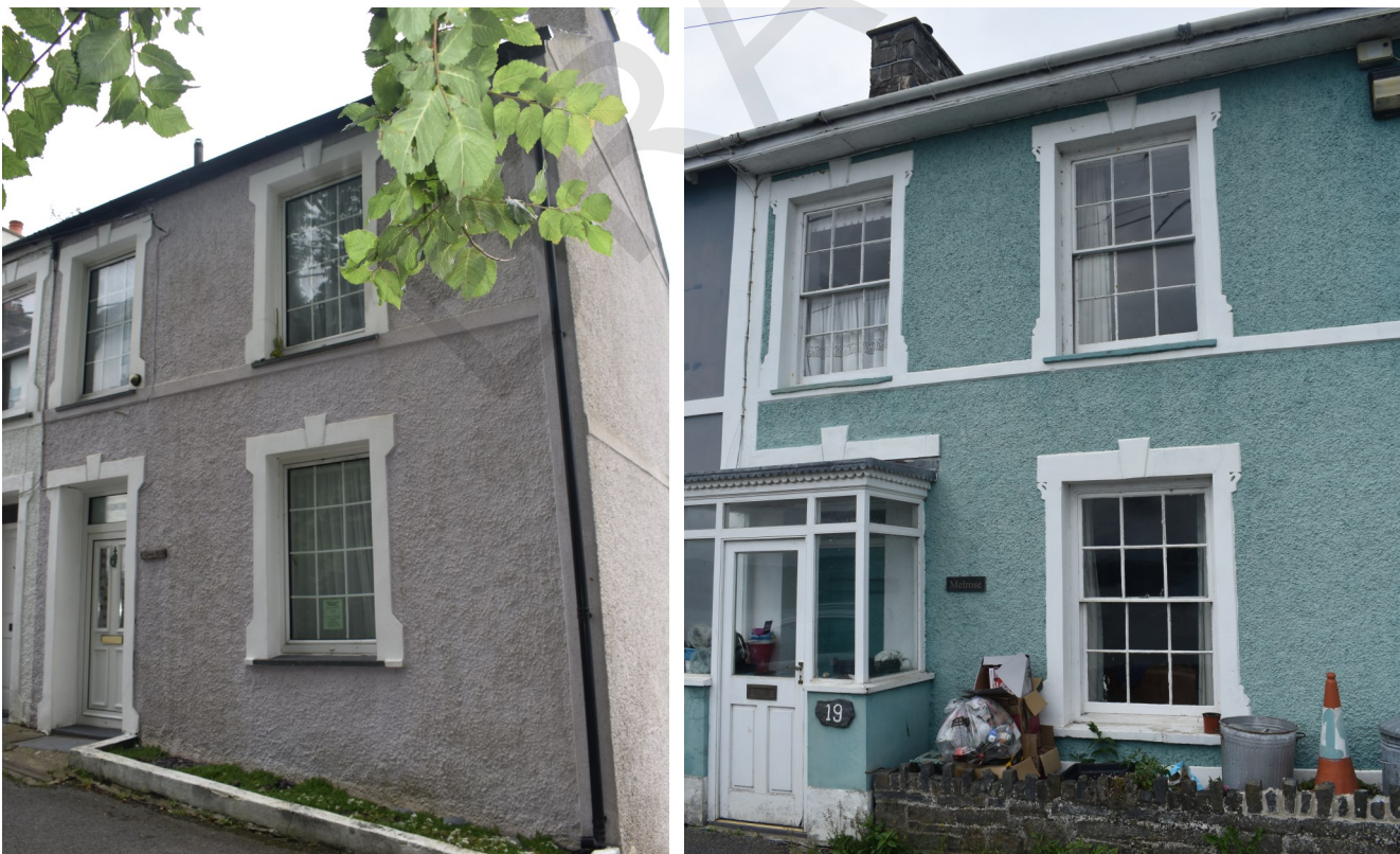
Figs. 1 and 2 Two houses of similar ages, demonstrating the visual impact that inappropriate replacement windows and doors can make on the character of a building
